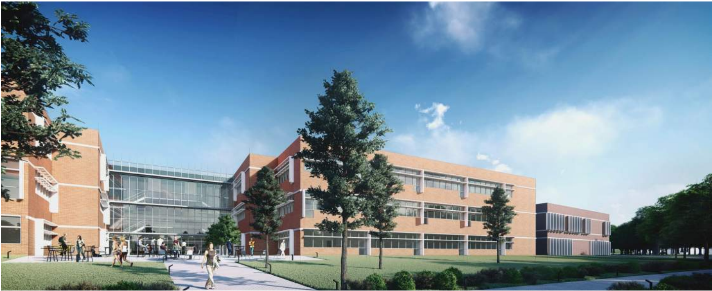
View of eastern classroom wings
